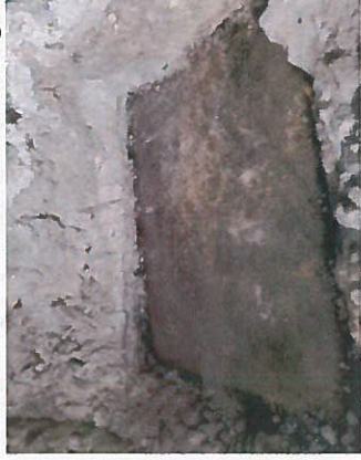
R-5 Vault after excavating
